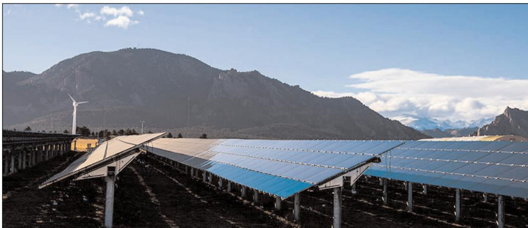
**CdTe solar cells are the second-most-common photovoltaic technology after silicon solar cells. CdTe solar cells rely on a thin film of material to absorb light and convert it into electricity. Photo by Dennis Schroeder, NREL.**
